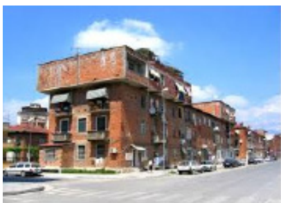
FIGURE 3: Additional unauthorized top of an existing building 14
